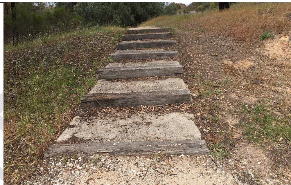
Image 16 – Timber & concrete stairs
